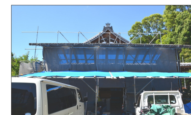
↑向拝の足場解体前
